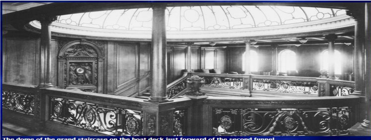
The dome of the grand staircase on the boat deck just forward of the second funnel.
